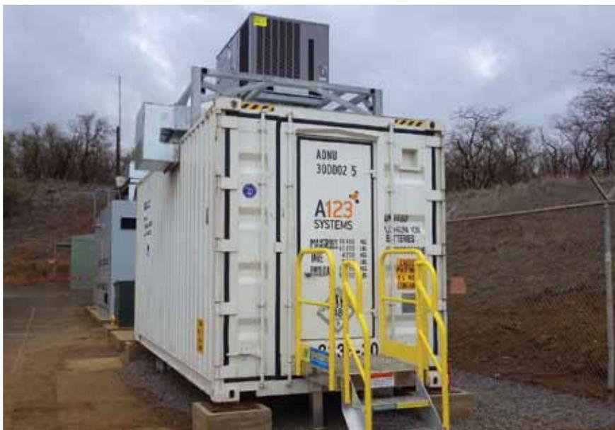
This 1 MW/1 MWh A123 lithium ion battery system at the Maui Electric Wailea Substation, Hawaii, began operating in May 2013. AES Westover and AES Laurel Mountain also use A123 systems. (Photo courtesy of A123 Energy Solutions)
